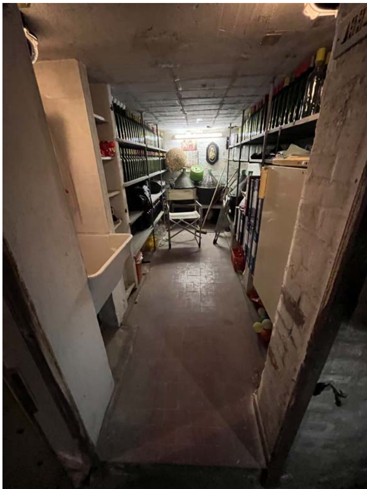
10. Cantina – Piano interrato
